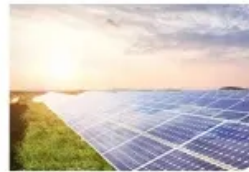
Energy Storage System
